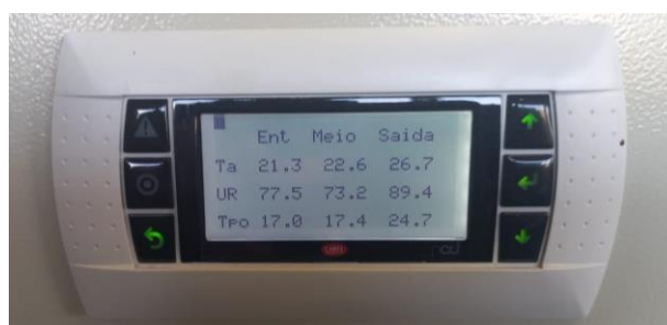
Figure 4: human-machine interface screen with temperature and relative humidity data: input (Ent), midpoint (Meio) and output (Saida).
